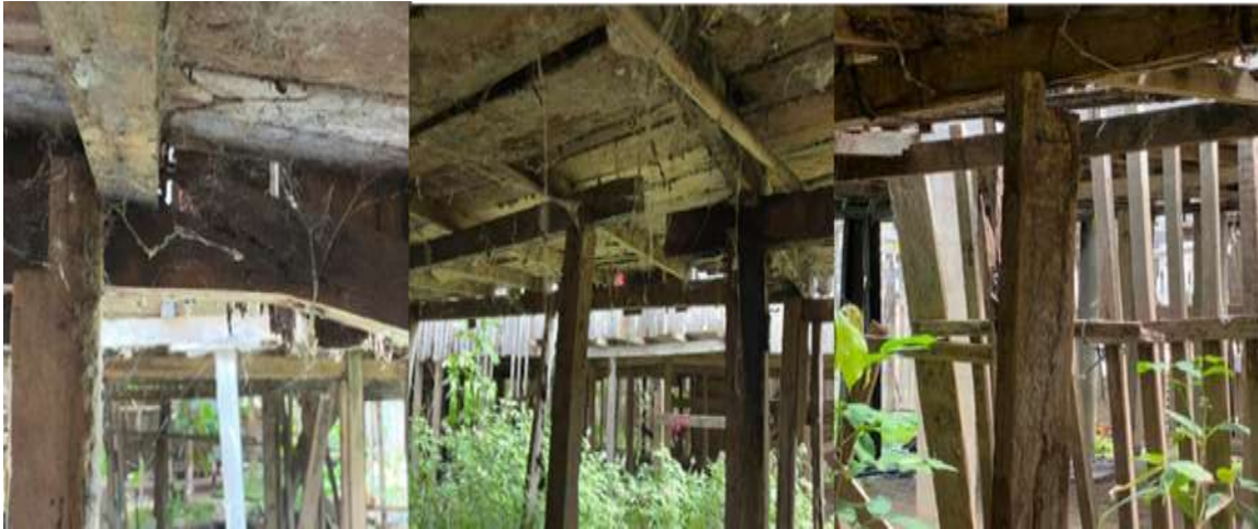
Fig. A2. Occurrence 2. Rupture/displacement in apparent structural elements. GUT score: 125
