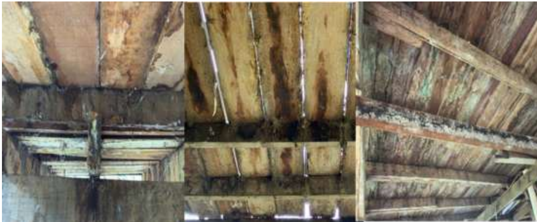
Fig. A7. Occurrence 7. Staining/mold fungi. GUT score: 80
