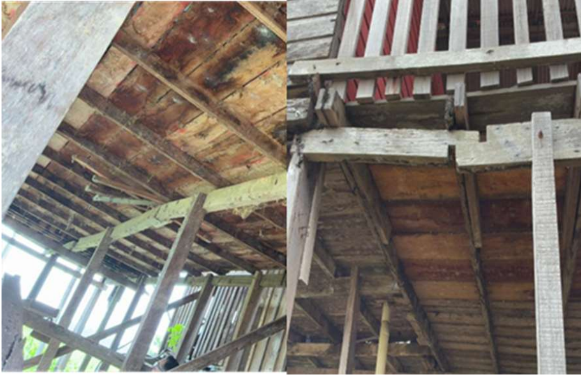
Fig. A4. Occurrence 4. Visible deformation in beams and pillars. GUT score: 125
