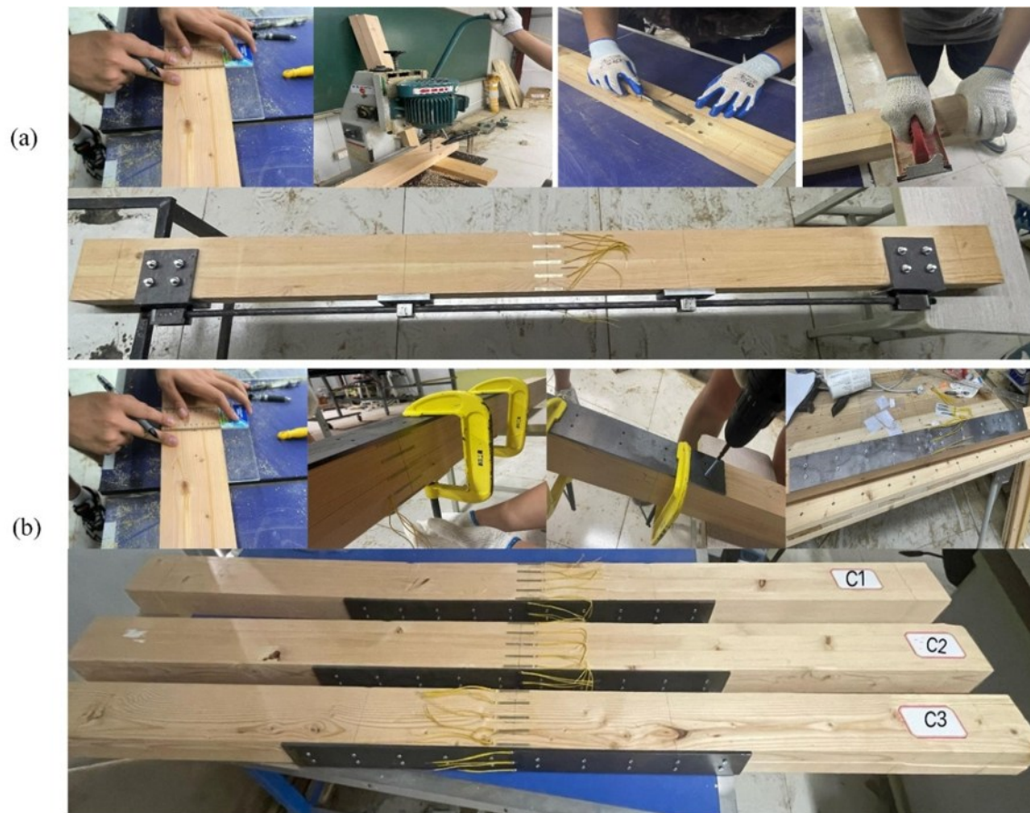
Fig. 3. Reinforcement process: (a) B series and (b) C series
