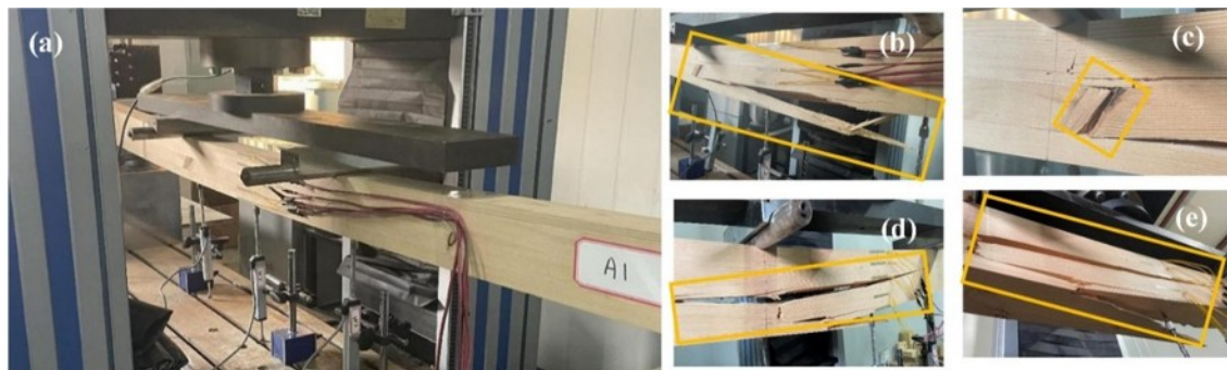
Fig. 5. Typical failure of unreinforced glulam beams
