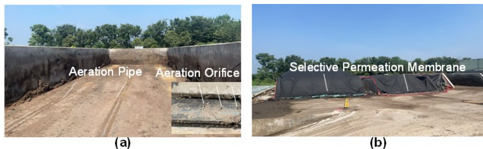
Fig. 1. (a) Empty composting tank body and (b) compost aeration process
