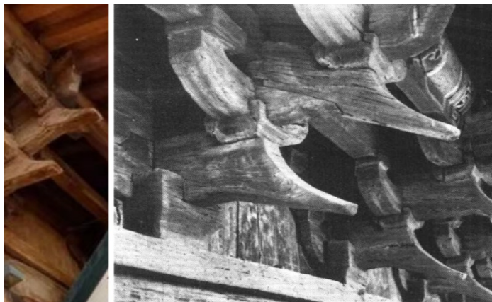
Fig. 2. Yanghe Tower's column cap and bracket
