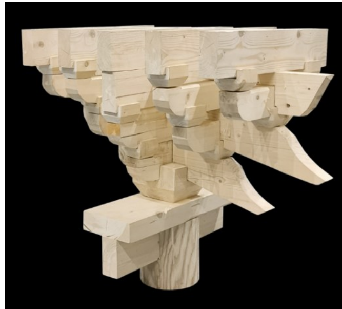
Fig. 3. The perspective drawing of experimental model for column-cap bracket sets of the memorial hall of Confucius
