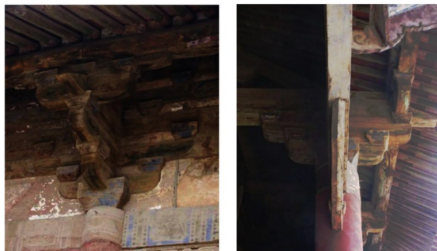
Fig. 2. The authentic Five-tier outer eave column-head Dougong bracket in the Dule Temple Gate
