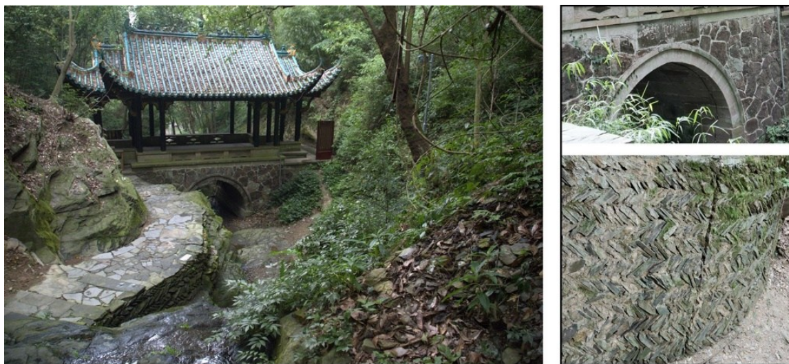
Fig. 1. General view (a) and stone materials of Yuxian bridge arch and abutment (b)
