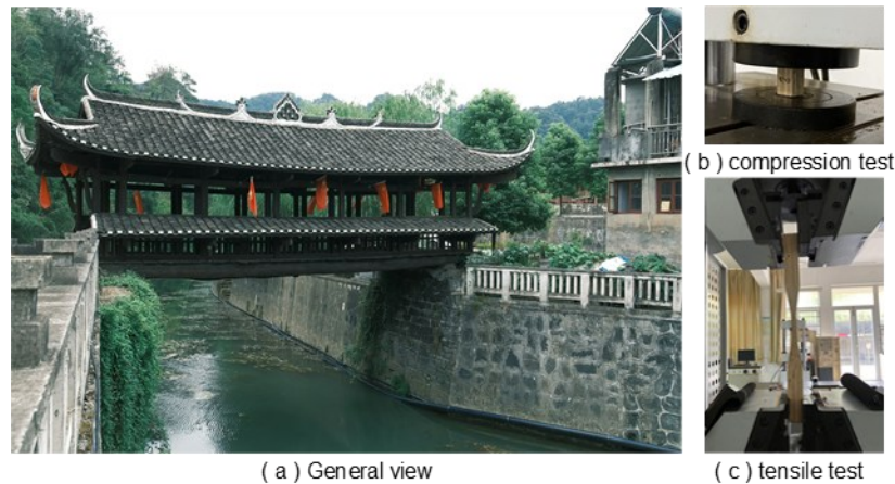
Fig. 1. General view and material tests of Yinjia bridge
