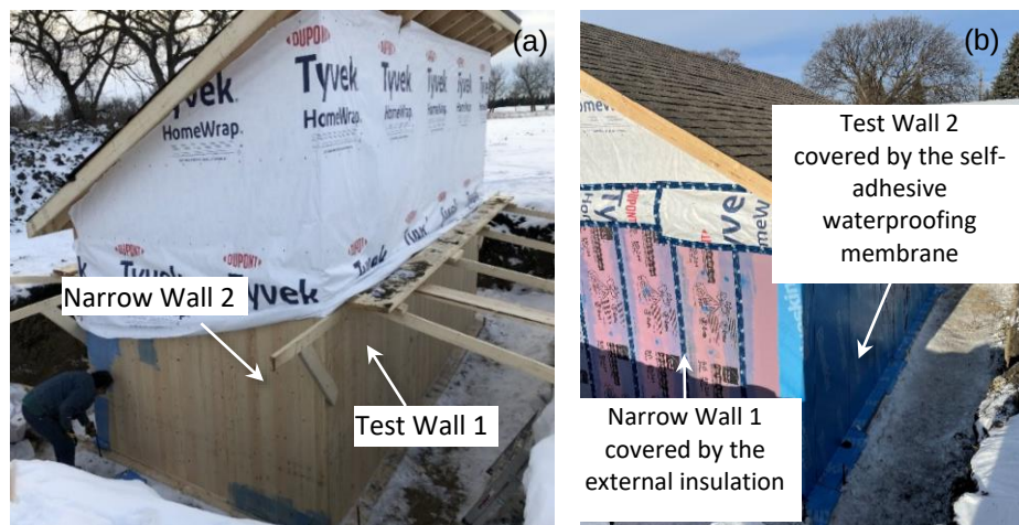
Fig. 3. CLT basement construction: a) applying fluid water protection to the CLT narrow wall 2 in November 2021, b) Test Wall 2 water protection in November 2021
