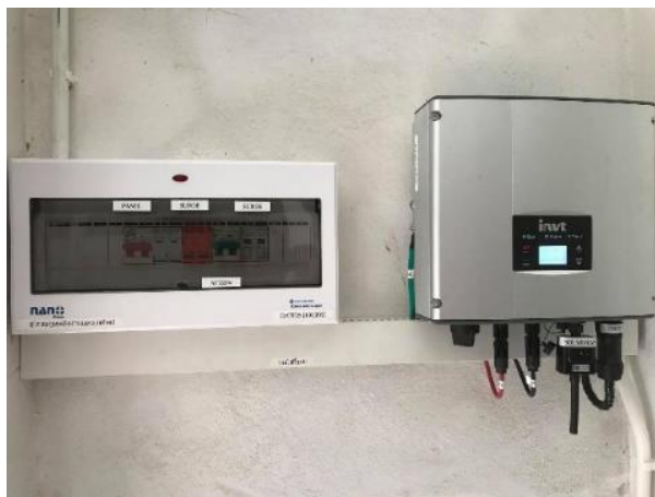
Fig. 2. The 3-kW grid-tied inverter can connect solar power to the hydraulic compression molding machine
