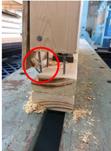
Fig. 9. The studs separated from the bottom beam of the shear wall connected by twist nails
