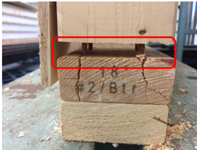
Fig. 7. The pull out of the studs
